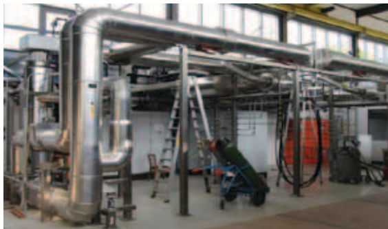
Picture of the Helium Low Pressure Loop at Karlsruhe (HELOKA-LP) that will be used to validate the High Flux Test Module thermo-hydraulic characteristics
