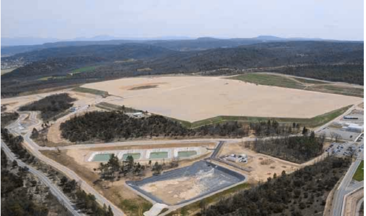
An aerial view of the ITER construction site in Cadarache, France (Image courtesy of Agence ITER France)
