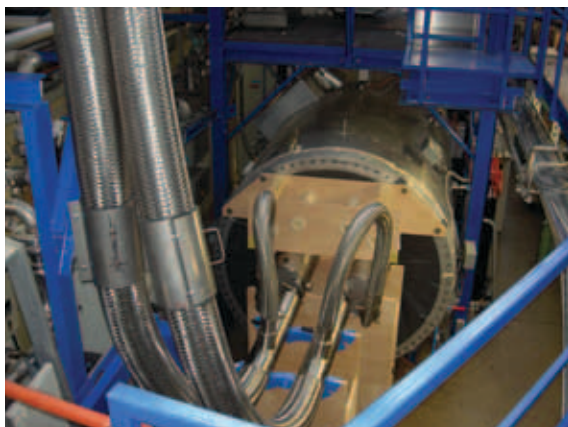
View of TIMO-2 Facility at KIT being upgraded to provide 4.35 K supercritical He for testing the ITER Torus Cryopumps (Image courtesy of KIT)
