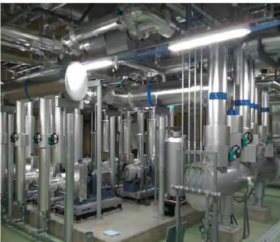
Cooling system for the Helios supercomputer.
