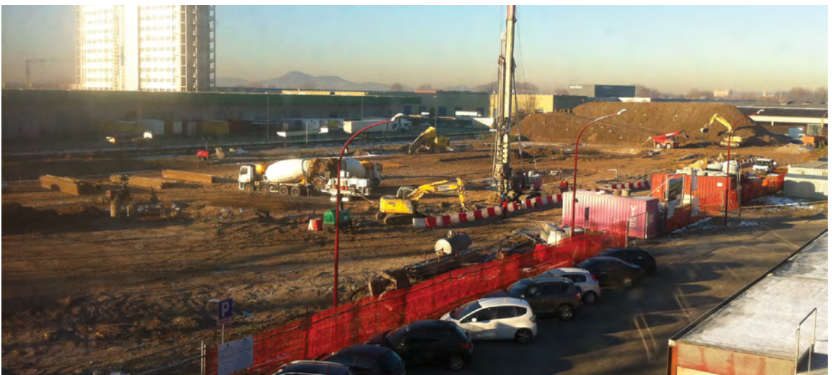
Neutral Beam Test Facility building construction
