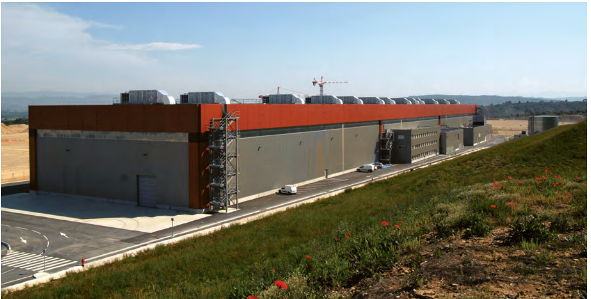
External view of the poloidal field coils building
