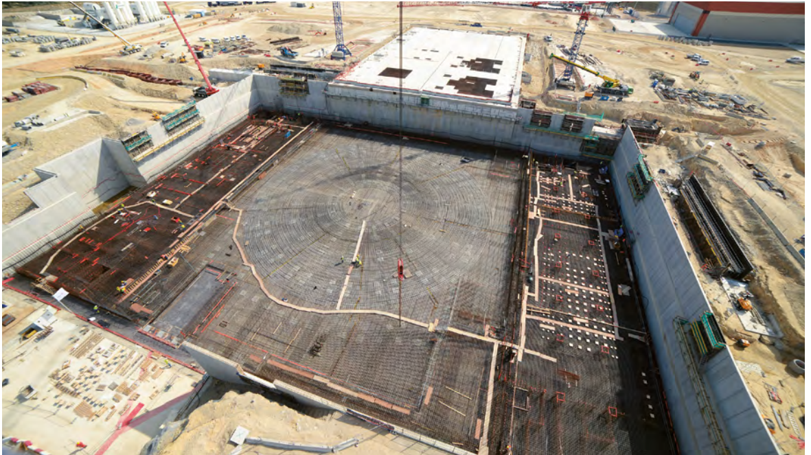
Tower crane view of the F4E work site: Tokamak Complex Reinforcement, Assembly Hall Foundation slab in the background
