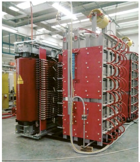
RF Power Supplies for ISEPS of SPIDER at OCEM Energy Technology premises
