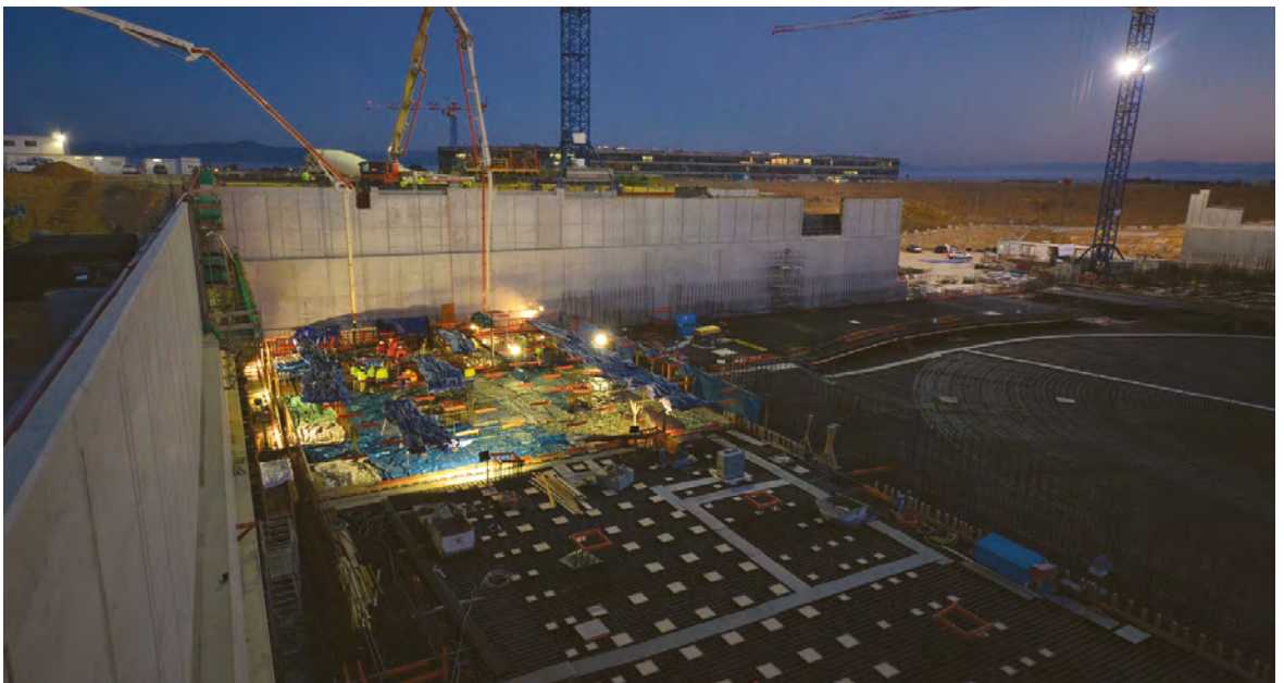
Pouring of first concrete to B2 slab of Tokamak complex 11 December 2013 (B74 Diagnostic Building)
