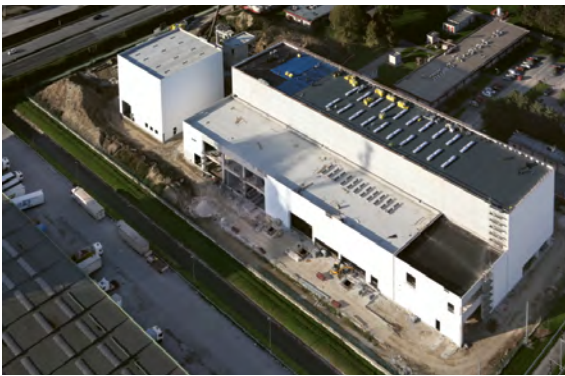
PRIMA building erection at Padova site (Consorzio RFX premises)
