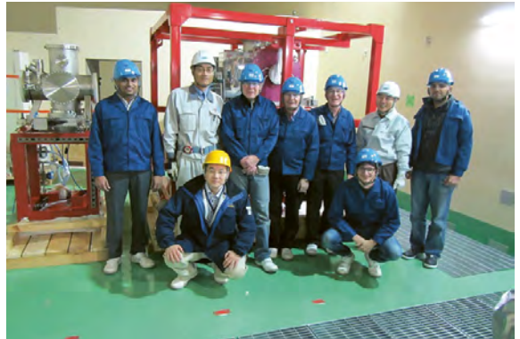
Pre-installation of the injector components at the LIPAC hall by members of the LIC unit formed by PT, JA-HT and EU-HT members
