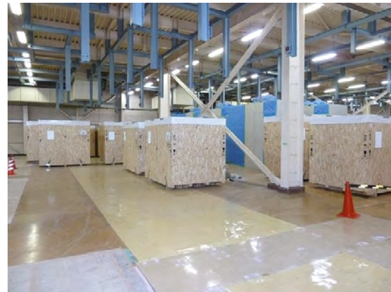
QPC components stored in the rectifier building
