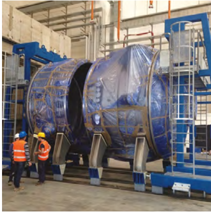
SPIDER vacuum vessel installation at NBTF
