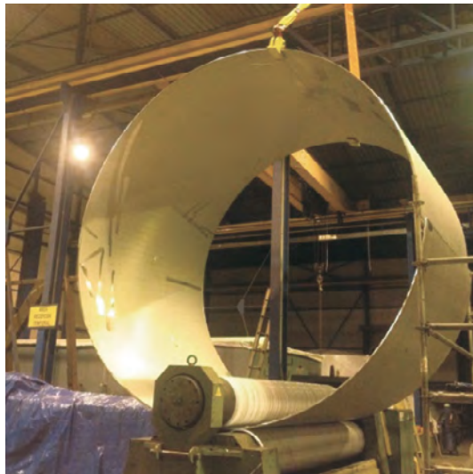
Cold forming of 100 m³ tank shell sector.
