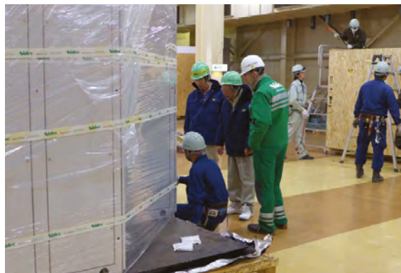
QPC on-site installation activities
