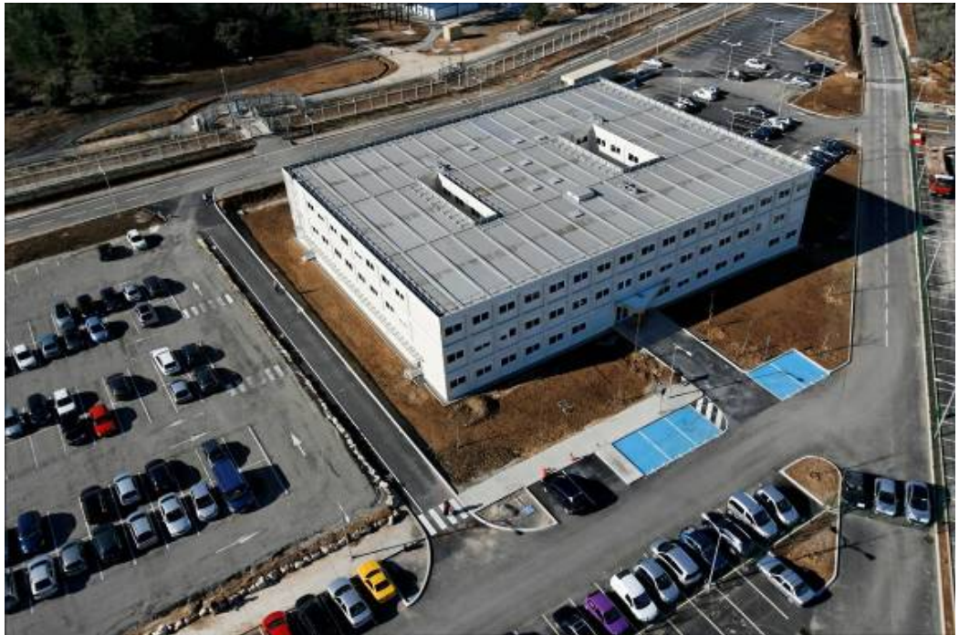
Figure 11 - Temporary ITER Headquarters Nov 2008
