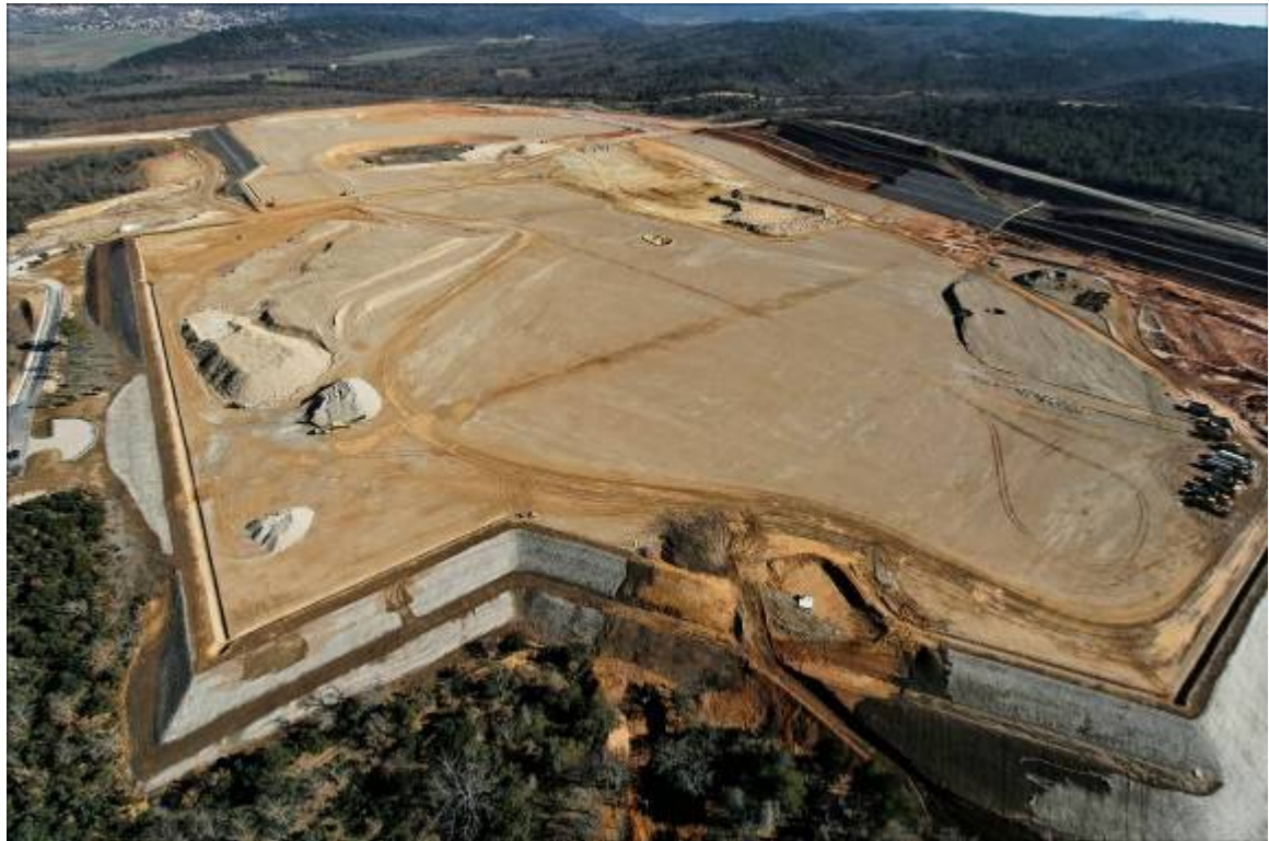
Figure 10 – ITER Platform end of 2008
