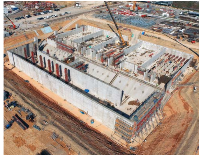
Civil engineering works progressing at the water basin and cooling water stations of the ITER device, April 2017, © E. Riche/ITER Organization
