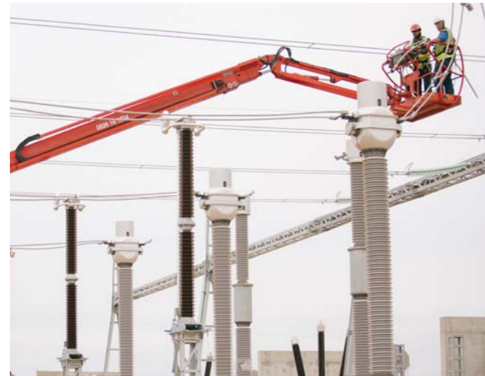
Technical teams checking the cabling where the ITER substation will be connected to France's grid to receive 400 kV, November 2016, © LNM
