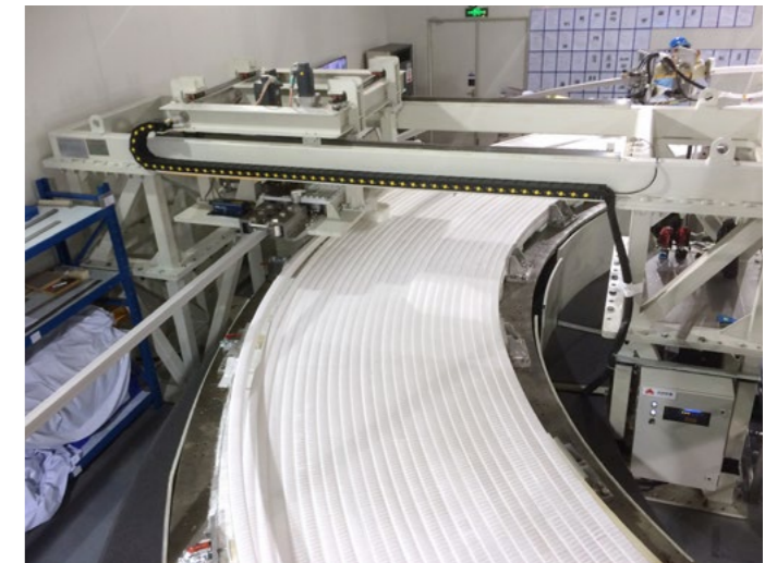
The Winding of the first Double Pancake of Poloidal Field coil 6 has been completed, ASIPP, China
