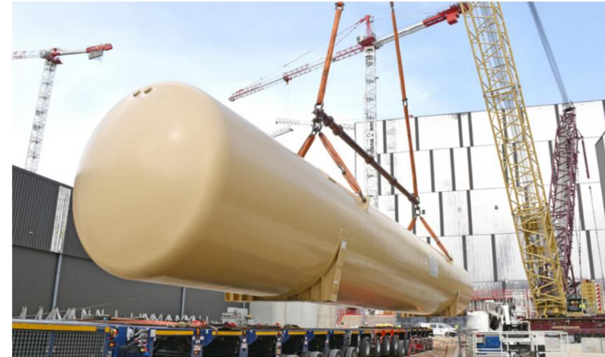
Lifting one of the two quench tanks financed by F4E and produced by Chart Ferro. ITER Cryoplat, April 2018.
