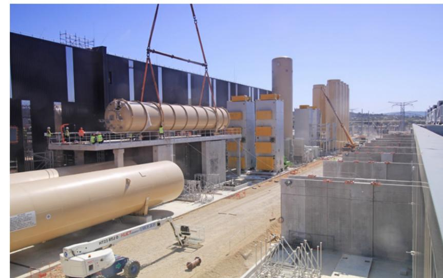
More components produced by Europe have been installed on-site: the two quench tanks on the ground, the LHe tank on the level above, and the cold boxes. At the far end the remaining cryogenic tanks.
