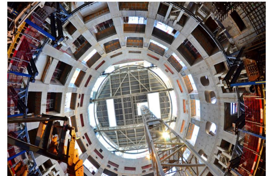
View of the ITER Bioshield lid, positioned 30 m high, ITER construction site, Cadarache, March 2018 © ITER IO
