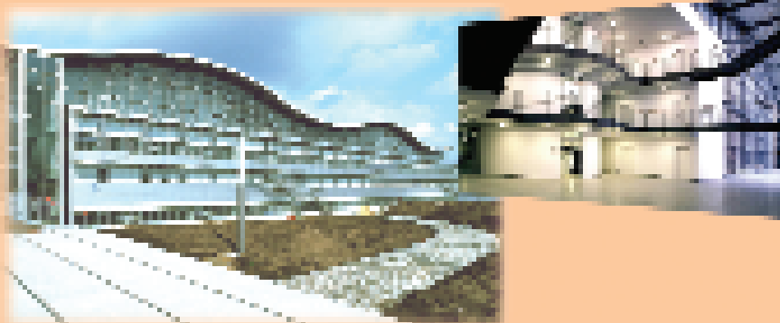
IPP building (Wendelstein 7X) in Greifswald - D
