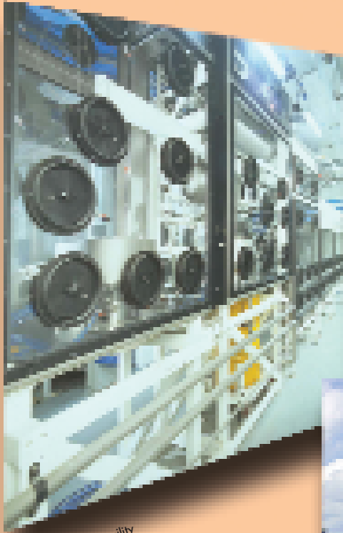
Tritium Handling Facility
